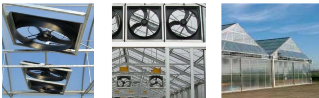
Figure 17 Roof and axial fans of Thermo-System™, ( www.parkson.com )
