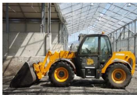
WWTP Palma de Mallorca, Spain ( www.parkson.com )
