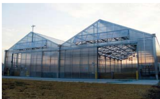
Figure 15 Thermo-System installed in Okeechobee, Florida, USA ( www.parkson.com )
