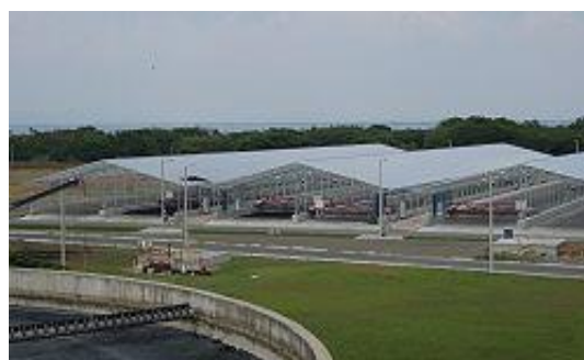
Figure 16 WendeWolf system installed in Managua, Nicaragua ( www.wendewolf.com )
