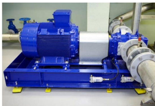
Figure 2 Pressure Reduction Turbine (Source: www.zeropex.com )
