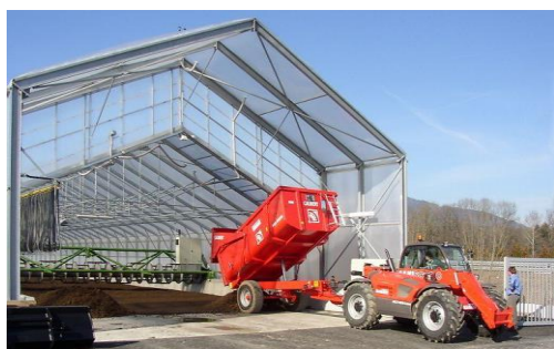
WWTP Reignier, France ( www.wendewolf.com )
